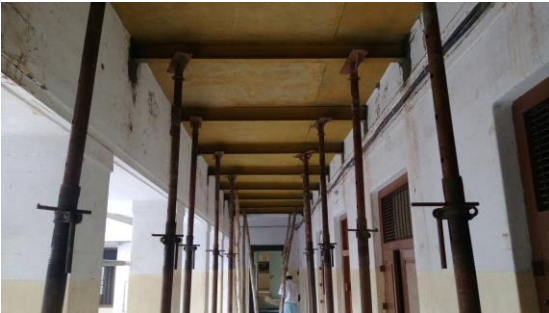
Main Block corridor – under construction
