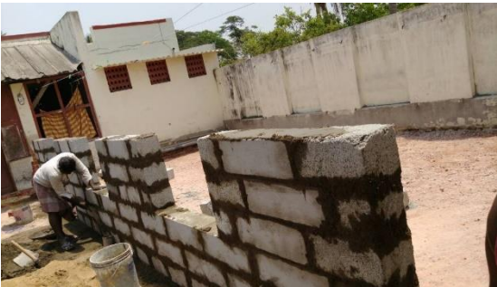
First floor new rooms under construction
