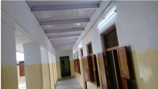
Main Block corridor – after renovation
