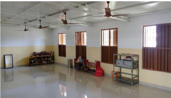
New rooms after refurbishing
