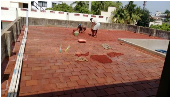
Waterproofing on the second floor
