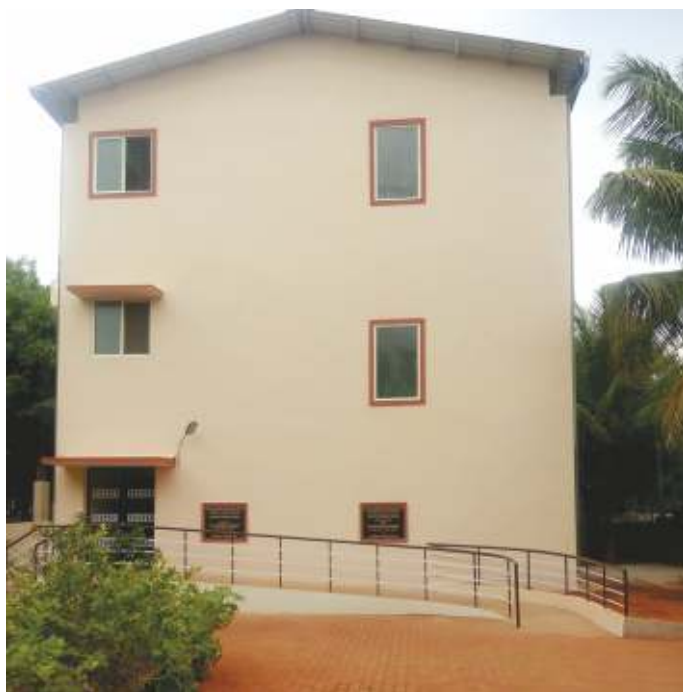
New Nagercoil building
