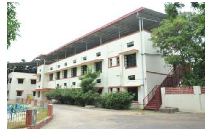
Infant and Toddler Block after renovation
