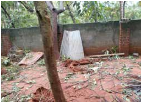
Damage caused by Cyclone Ockhi
