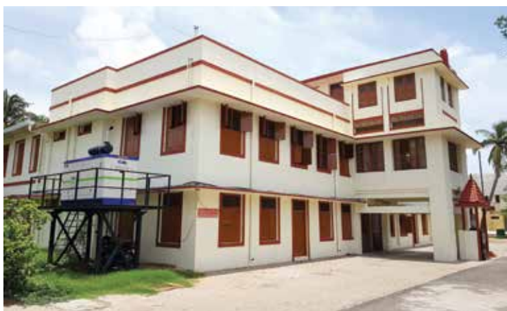
Outer view of the renovated Main Block
